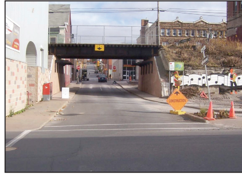
Large diameter corrugated HDPE pipe was buried underneath roads in New Glasgow for its CSO Project.
