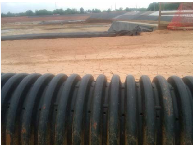
Corrugated HDPE pipe with a Class II perforation pattern enables water to enter the long-life system and be conveyed to a central collection point.
