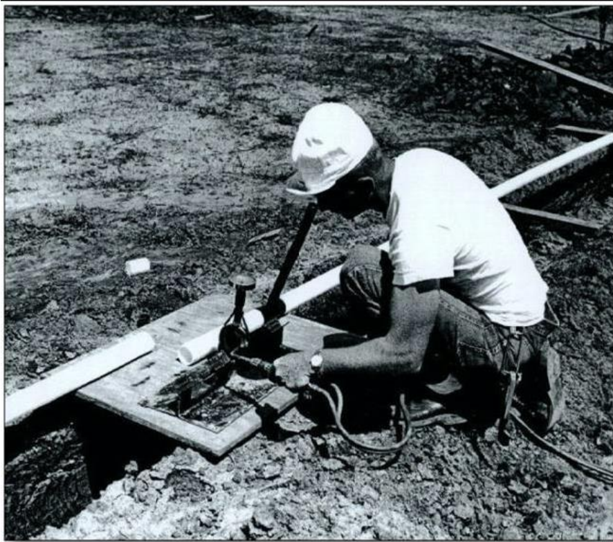
Figure B1 - Natural Color Polyethylene Pipe being Fused, 1959, in Caney, Kansas
