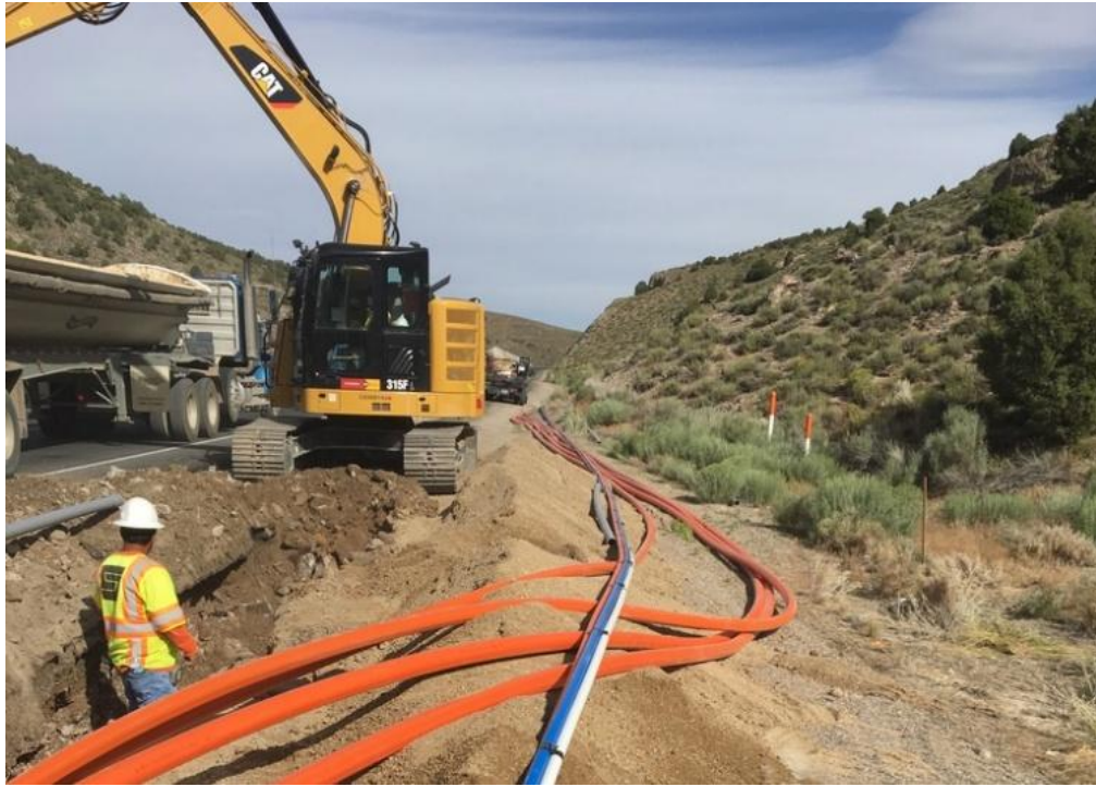
Figure 20 - Conduit being laid flat before installation.
