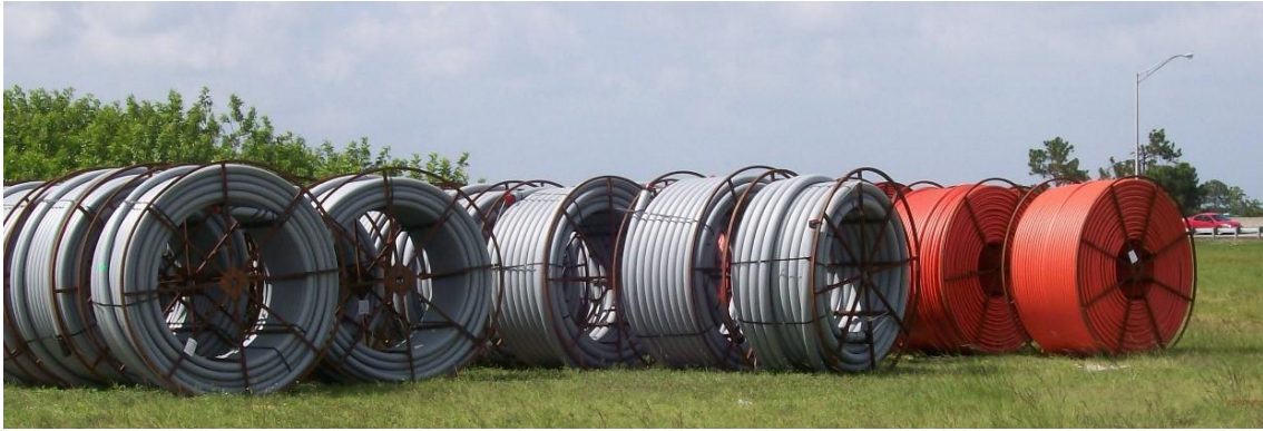
Figure 8 - Reels stored vertically on flat, level jobsite.
