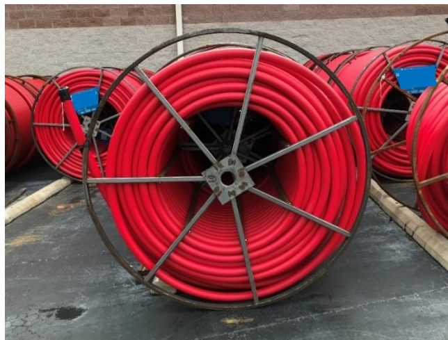
Figure 7 - Reels stored vertically on jobsite. Note curbs to prevent rolling.
