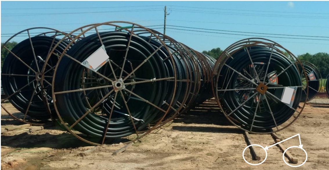
Figure 9 - Reels stored vertically on flat, level jobsite with lumber chocks.
