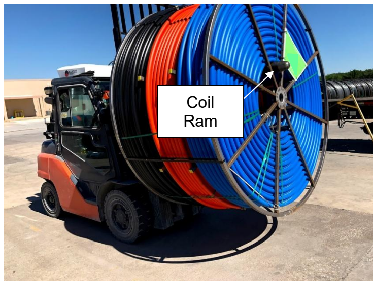
Figure 6 - Lifting a reel with a coil ram. Note ram end passes all the way through coil/reel.
