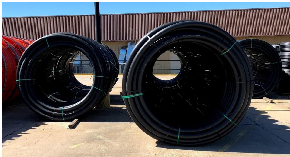
Figure 15 - Coils stored vertically on flat, level jobsite with lumber chocks.
