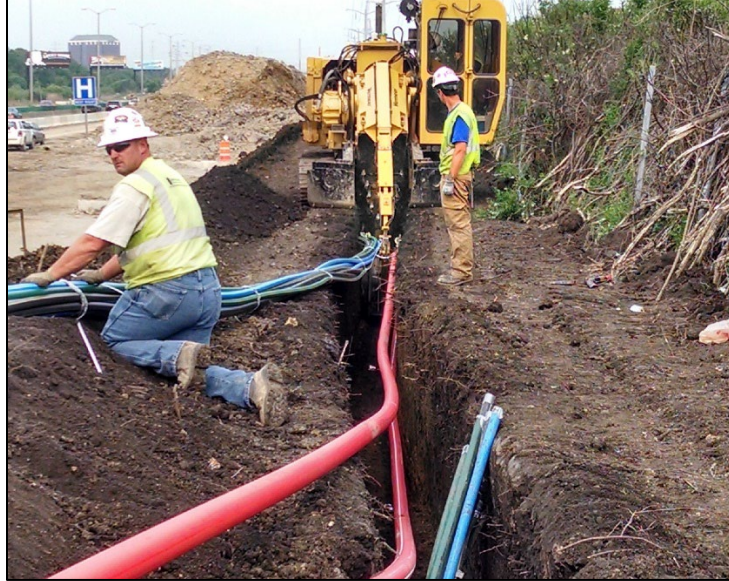
Figure 1: Open Cut Continuous Trenching Installation of HDPE Conduit
