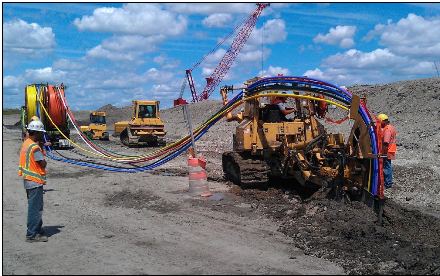
Figure 2: Plowing Installation of HDPE Conduit
