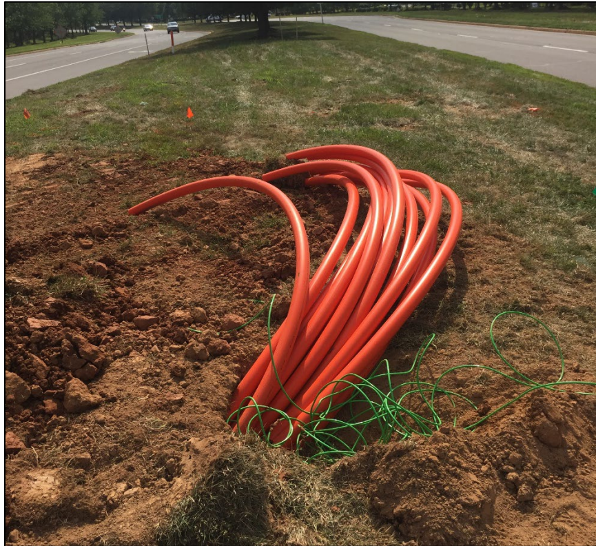
Figure 3: HDD Installation of HDPE Conduit
