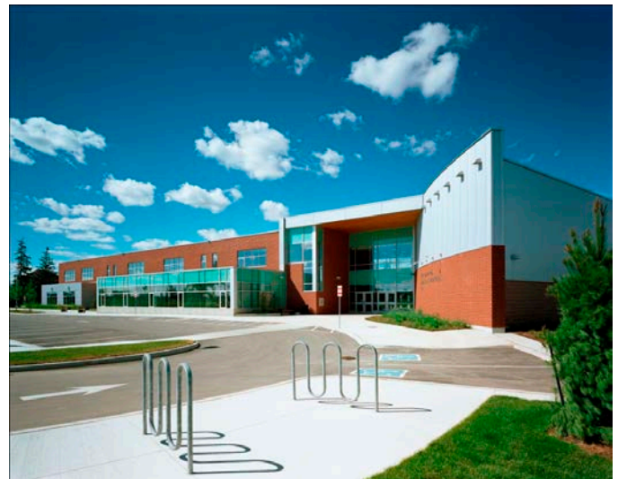
JSF High School features a REHAU radiant slab heating and cooling system installed throughout the building. Photo © Patrick Kennedy
