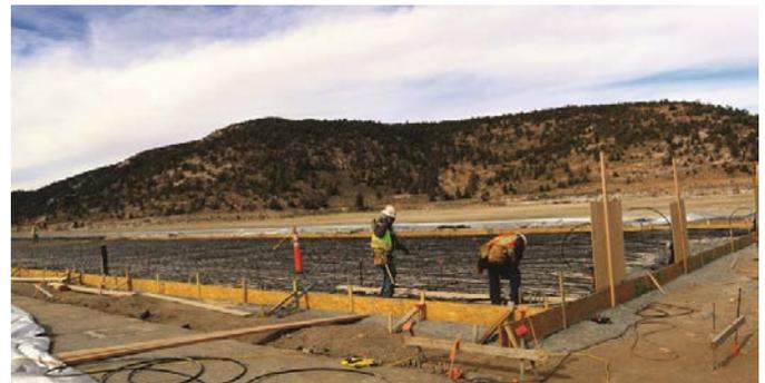
Some 22,500 linear feet of Viega PEX Barrier tubing was installed in less than one day using Viega Climate Mat.
