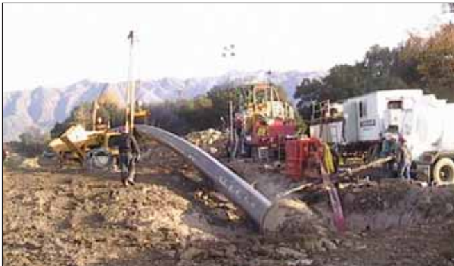
A 30" steel casing, pulled through 48" surface casing into the hole.
