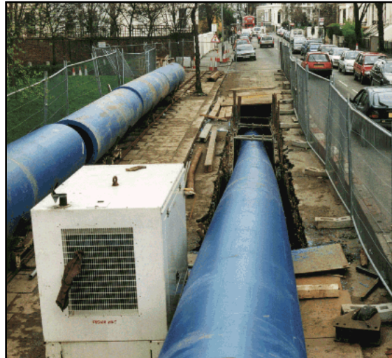
Fig 1. Renovating an old iron water main using large diameter PE pipe
