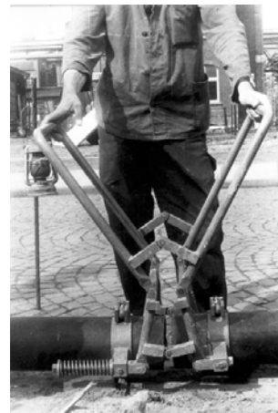
Fig. 9. Manual application of joining pressure in hot plate butt fusion process
