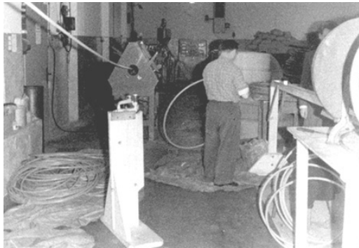
Fig. 10. Production of Hula Hoops at Gröter in Emsdetten (by courtesy of egeplast)
