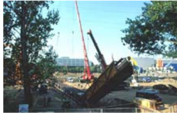
PE 100 filament wound pipes for a culvert (pipeline under river, 2003)
