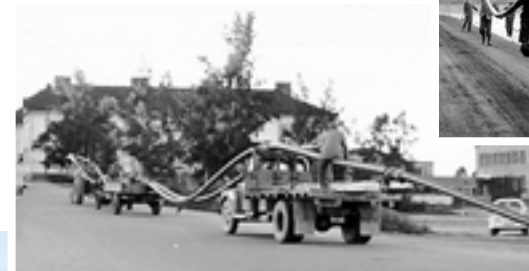
Unconventional method of transporting pipes to site
