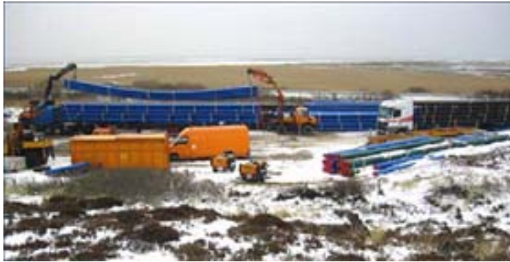
Laying of pipelines for drinking water and gas (Island of Sylt, 2005)
