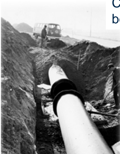
Laying of underground pipes for industrial sewage (Frankfurt 1963)
