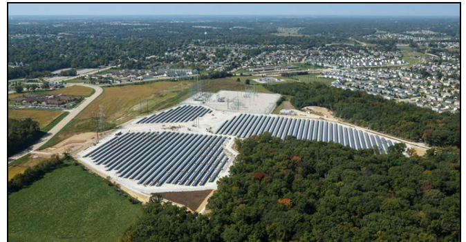
The O'Fallon Renewable Energy Center encompassing approximately 20 acres in O'Fallon outside of St. Louis. With 19,000 solar panels, it is one of Missouri's largest photovoltaic solar fields and is now generating 5.7MW of electricity enough to power 650 average sized homes.
