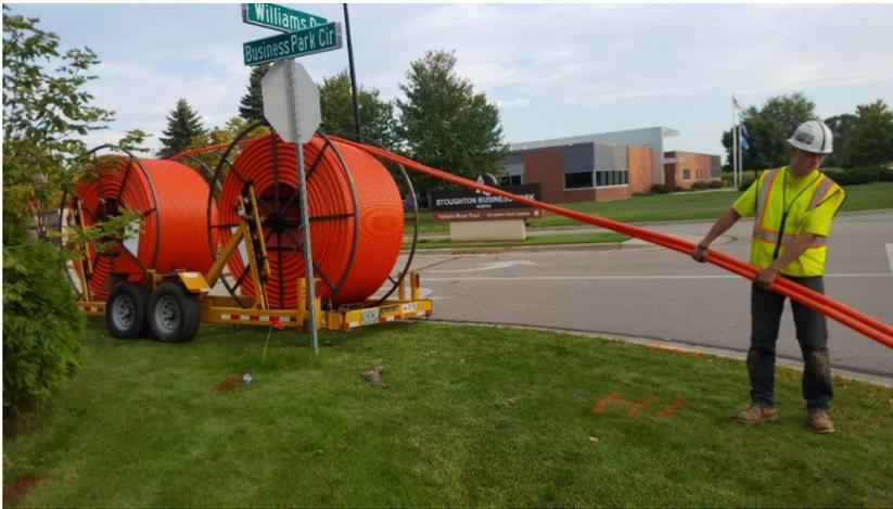
Teel conduit is being installed across Alliant’s service area in Iowa and Wisconsin to improve its telecom network’s security, speed, and reliability. For a utility with a large service area including more than 970,000 electric and 420,000 natural gas customers, reliability and capacity are crucial during critical events. The conduit will protect the existing infrastructure and allow for later expansion of network capabilities while providing cost savings to Alliant Energy.
