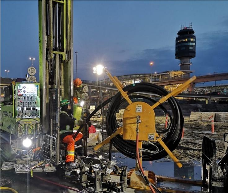
The Vancouver International Airport's new Central Utilities Building (CUB) will improve efficiency by centralizing all of the equipment needed to meet the airport's heating, cooling and electrical demand. To achieve this goal, the project will rely on one of the largest Geexchange systems in Canada. Geexchange technology uses the earth's renewable energy, just below the surface, to heat or cool buildings. This system will provide sustainable heating and cooling for the terminal.
