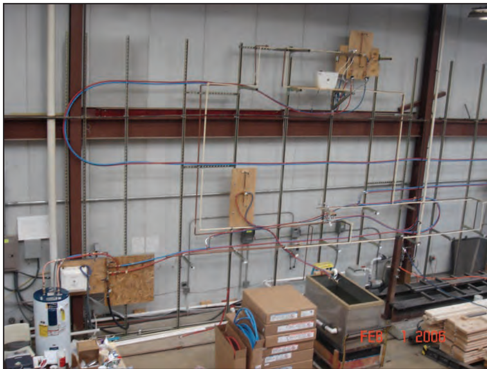
Figure 8.2 – Laboratory Test Set-up with Five Outlets, Hot Water Tank, and T&B System
