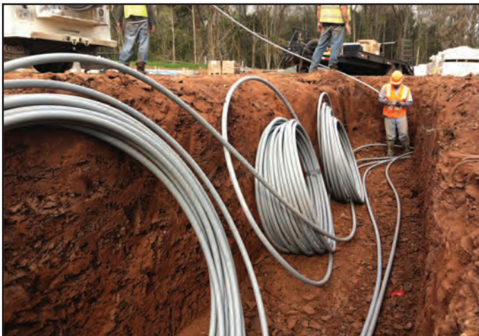
Figure 11.7 – PEX Piping in a Geothermal Application
