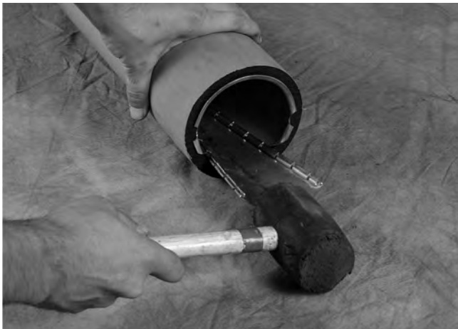
Figure 12 Install Split Ring Stiffener in PE Pipe
