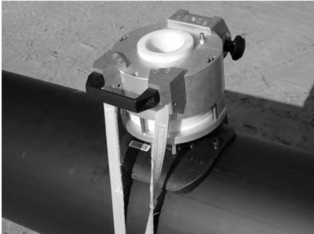
Figure 4 Electrofusion Patch Repair
