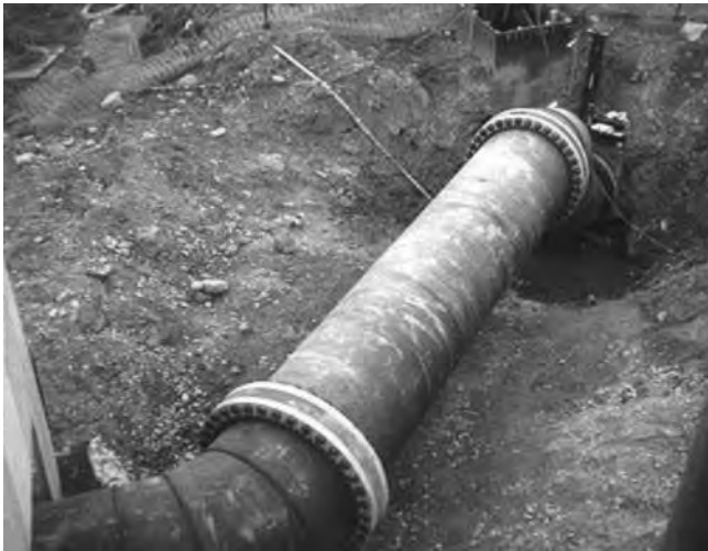
Figure 13 Flange Adapter Assembly
