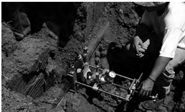
Figure 3 Saddle Fusion Repair
