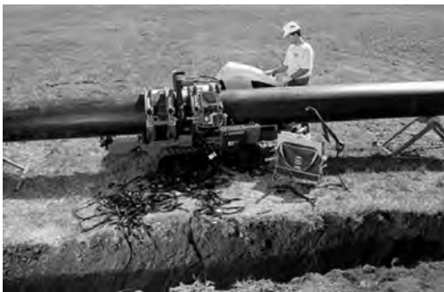
Figure 1 Above Ground Repair with Fusion Machine
