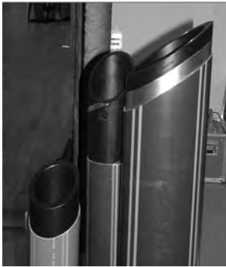
Figure 22 Protecting the PE Pipe from Shards
