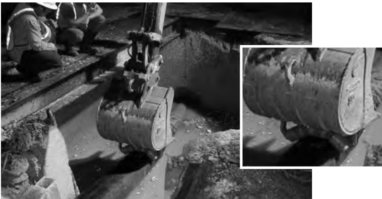
Figure 23 Protecting the PE Pipe from Grooves Using Welded Wheels on the Bucket
