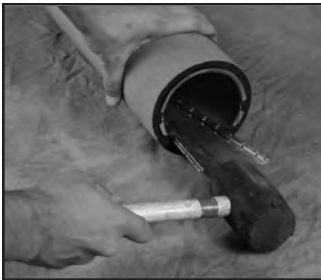
Figure 19 Install Split Ring Stiffener in PE pipe
