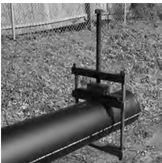
Figure 15 Mechanical Re-Rounding Clamp Installed
